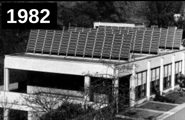
TISO 10 kW: 1° grid-connected PV system in EU
