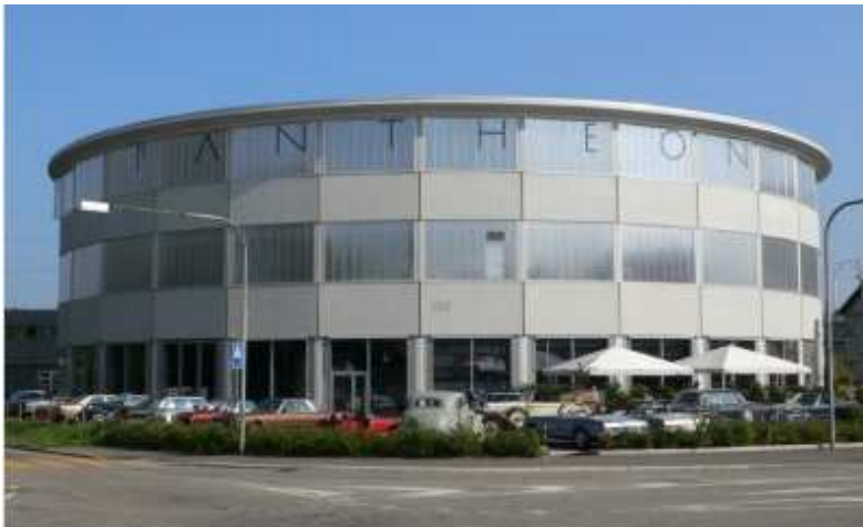
Intelligent efficient solid-state lighting 12.12.2016 in Muttenz
