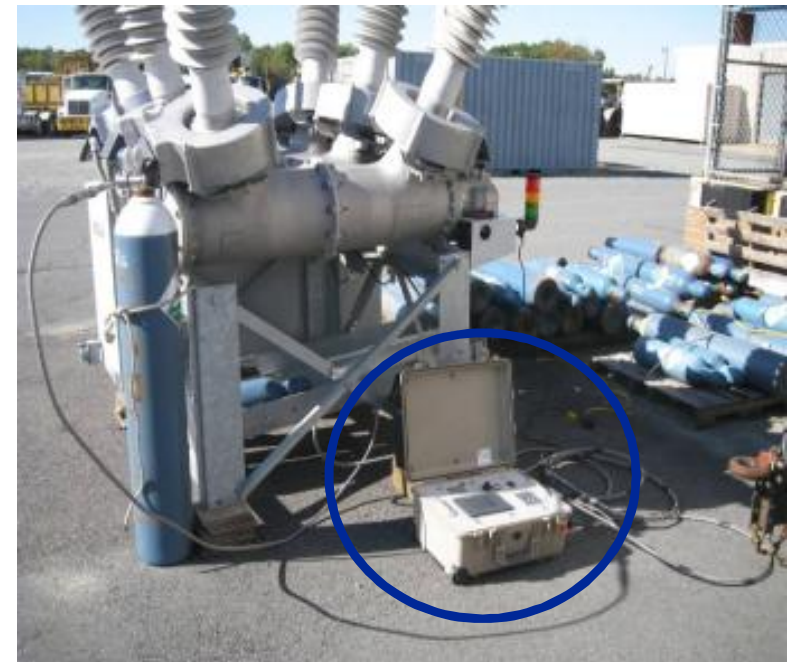
Gas analysis on a DTB, V. Williams, Company EMT
